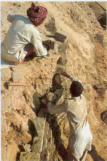
■ Figure 11. Temporary repair of eroded portions of the mosque using mud brick and clay/straw plaster, 1994
