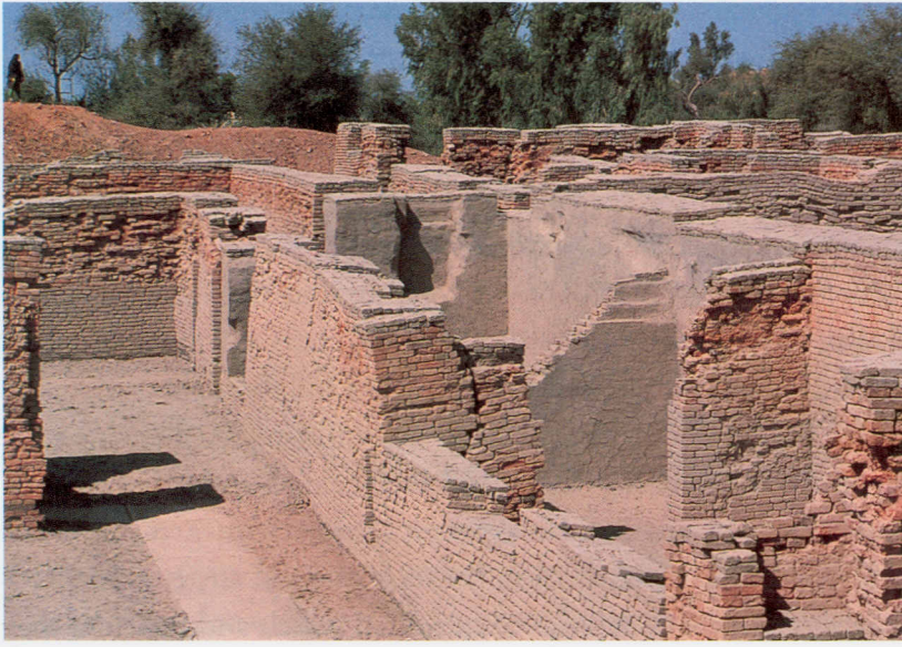
■ Figure 8. Vast expanses of brick architecture at Mohenjo-daro provide archaeologists with a more detailed understanding of the ancient city organization, but also require long-term conservation and restoration. These walls have been partly reconstructed, and a damp-proof course has been inserted to keep salts from percolating up through the structure. Some of the walls have been covered with clay and straw plaster to protect them from wind erosion.
