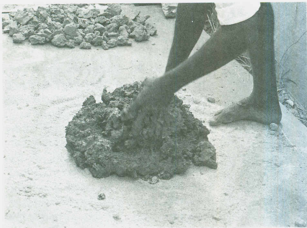
3 After the hard chunks of clay are compressed into smaller particles, water, sand, and rice husks are added to increase the workability range of the clay.
