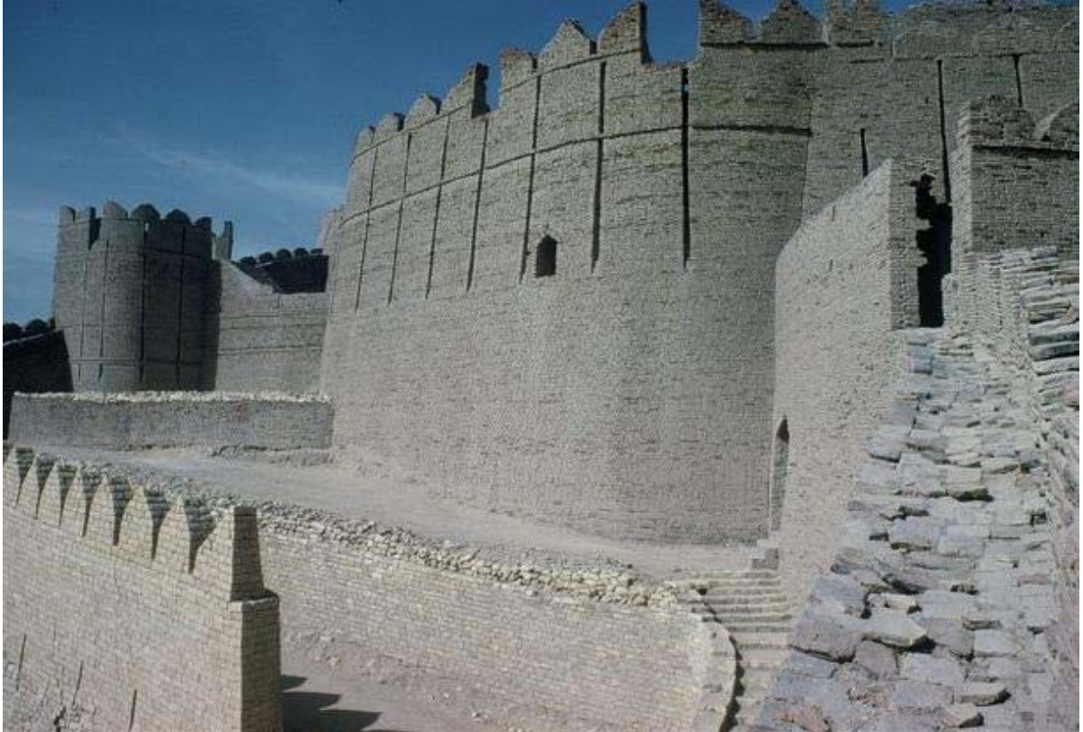
11. The walls and bastions of the Talpur's Kot Diji fort.
