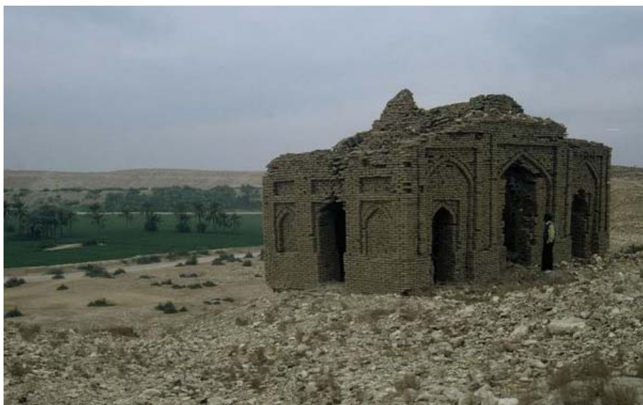
8. Aror: an unknown mosque, whose vault collapsed in the 1990s.
